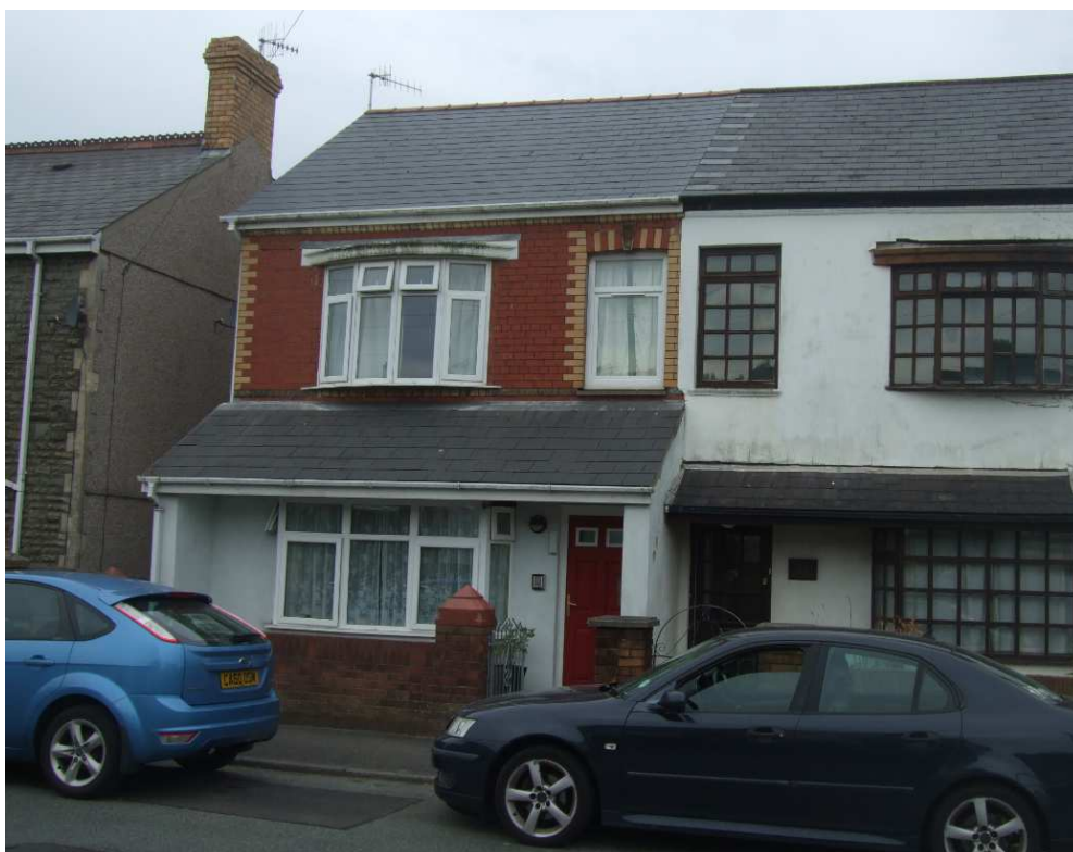
Figure 2 – Photograph of the application building (front)
